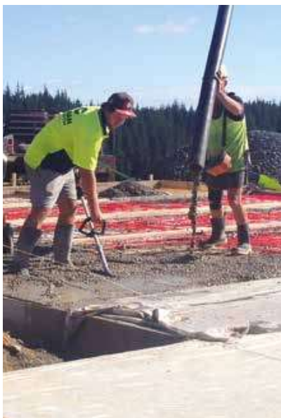
Above: The concrete pour stage of an underfloor central heating installation.
