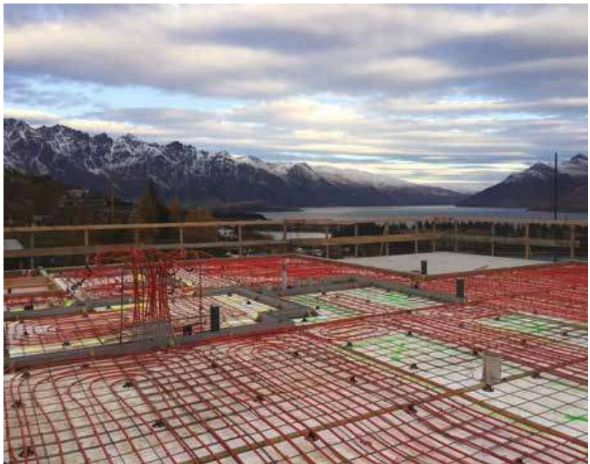
Above: A Queenstown underfloor central heating installation.
